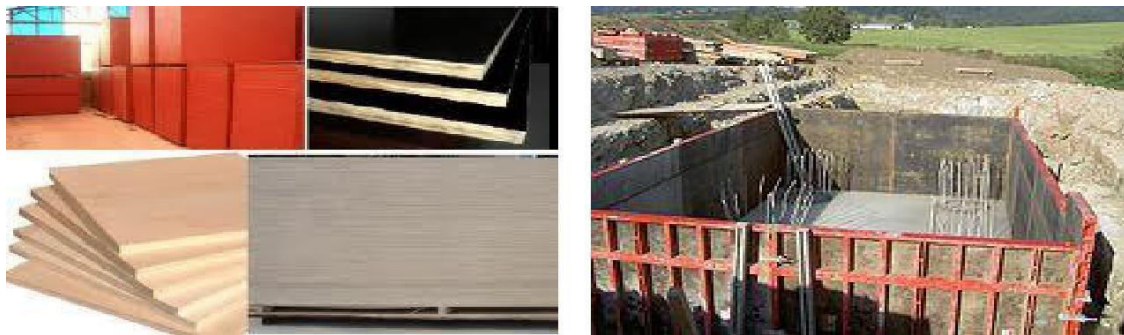
Formwork material (PLYWOOD) and Modular steel frame work
